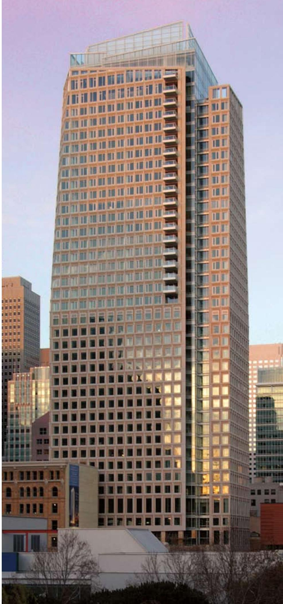
*The façade of the St. Regis Museum Tower in San Francisco features architectural precast concrete panels cast with two colors in each panel, with two levels of sandblasting used on each color in different areas, to create four distinct finishes.*
